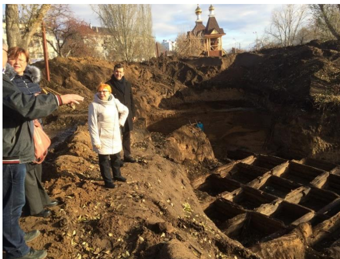
Figure 1: Underground structures of the XVIII century on Khlebnaya Square in Samara, excursion for the delegation from Latvia University of Life Sciences and Technologies V.Parsova and A.Celms.
