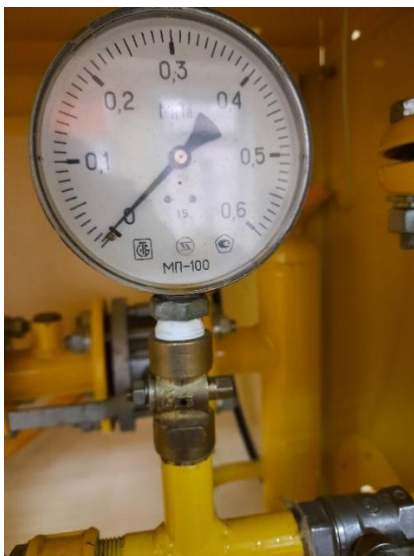
Figure 3. Installation of the manometer without lock nut
