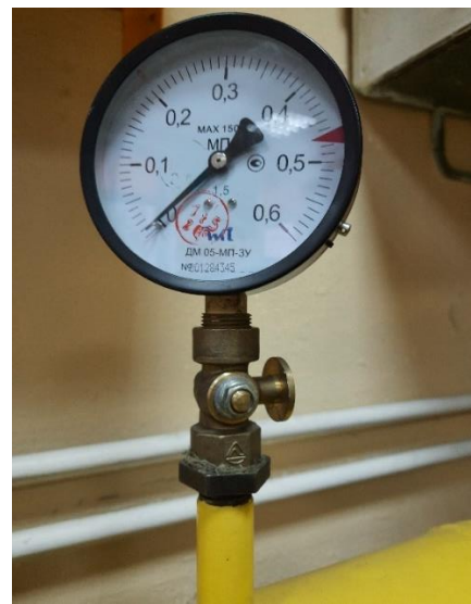
Figure 4. Installation of the manometer with a lock nut
