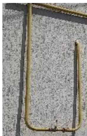
Figure 2. Scheme of the upper connection of the outer riser to the inlet gas pipeline with the location of the shut-off device on the horizontal section of the outer riser
