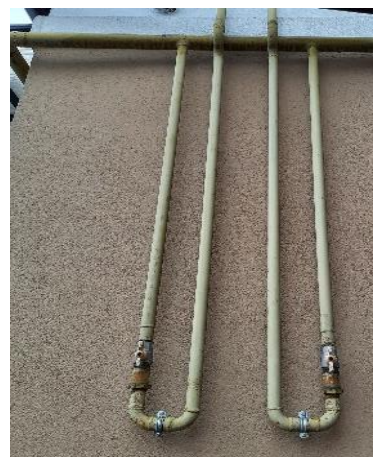
Figure 1. Scheme and photo of the lower connection of the external riser to the inlet pipeline with the location of the shut-off device on the vertical section of the external riser
