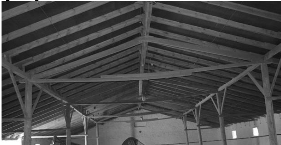
Figure. 1. Internal load-bearing wooden structures of grain warehouse No2
