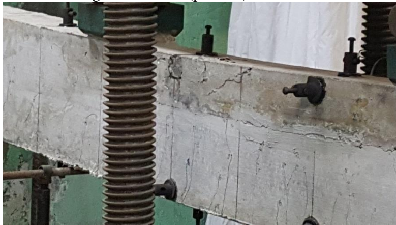
Photo 2. Partial destruction of the compressed zone of a reinforced concrete beam BOP-I-1
