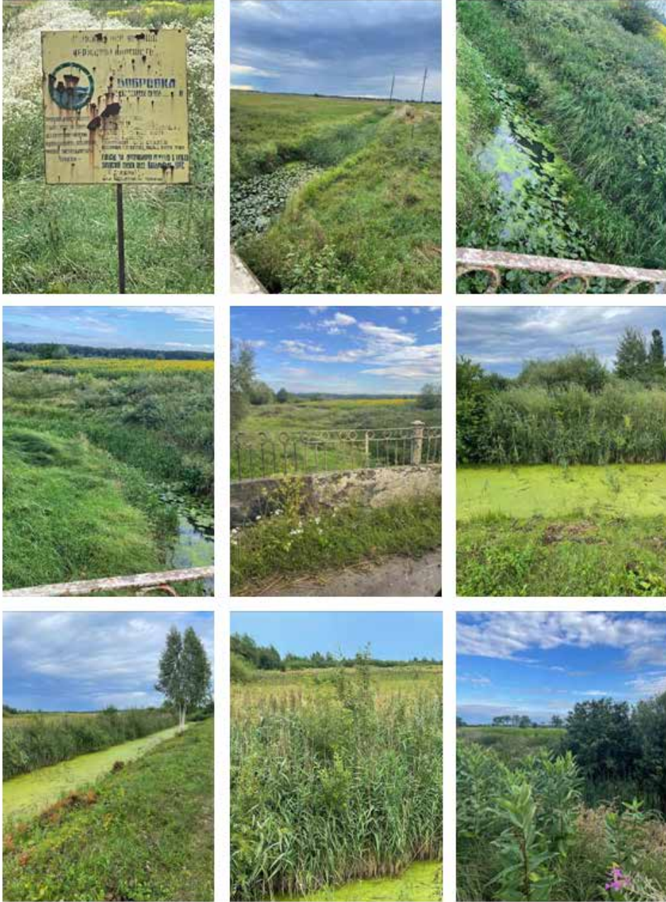
Figure 7. Condition of open channels in the “Bobrovka” drainage system
